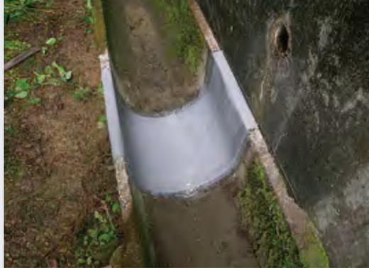
When compared to conventional mortar repairs, Catpad requires no mixing and is easy to apply without the need for specialist training. Once installed, it has a minimal curing time and can accommodate joint movement.
