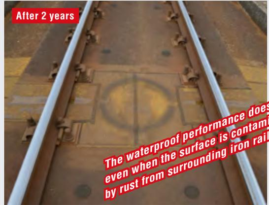
*The waterproof performance does not change even when the surface is contaminated by rust from surrounding iron rails.*
