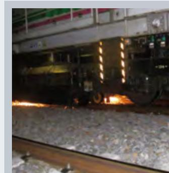
As part of ongoing maintenance rail grinding machines run to maintain the desired rail surface. Synthetic rubbers deteriorate due to sparks generated during grinding, but Catpad is hardly affected.
