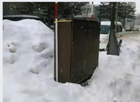
Prevents infiltration and freeze-thaw damage of street transformer base buried in snow for more than 3 months in winter.
