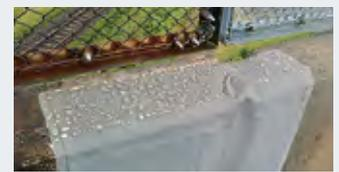
The water repellency of rainwater is maintained after three and a half years of construction.
