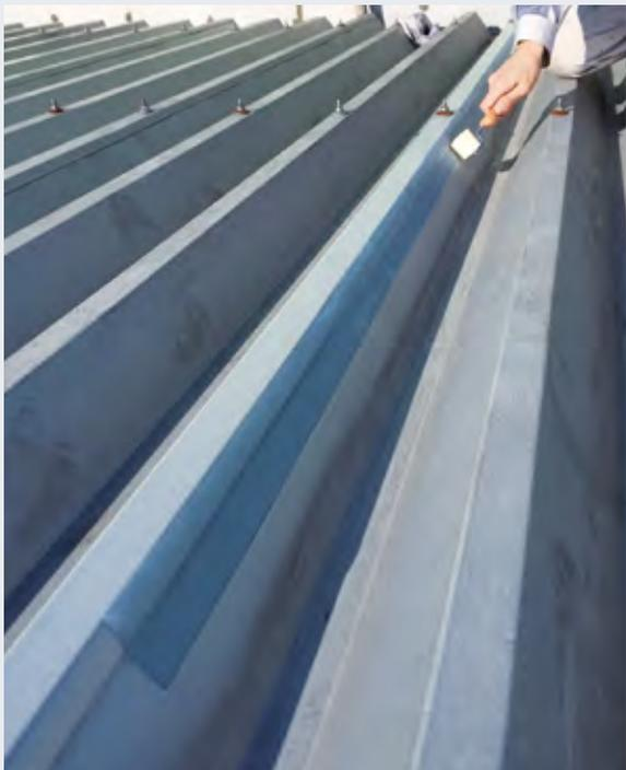
Immediately following its application, Catpad is able to accommodate movement and stop water ingress.
