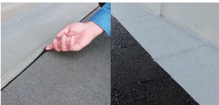
If this occurs, the outermost edges should be left unsealed. Catpad accommodates movement in a sideways direction.
