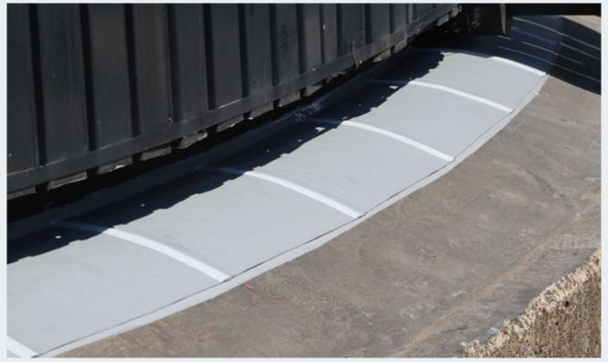
Shin-Etsu Silicone S COAT-57 has been used to eliminate low spots.
