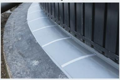
Catpad, Catpad-cloth and Cat-tape used to protect metal cover against corrosion.
