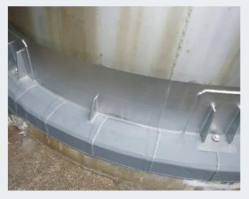
Catpad remains flexible even at below-freezing temperatures.
