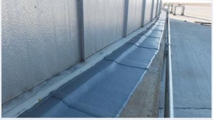
Foundation is mortar, so edges have been sealed using Sealant Master 300-G.
