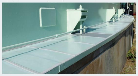
Installation in which Catpad partly covers the wall of the foundation for a small tank.
