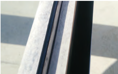
Remove masking tapes immediately after tooling.
