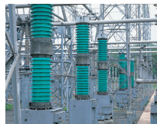
Protecting insulators from salt damage (application example for KS-63G)
